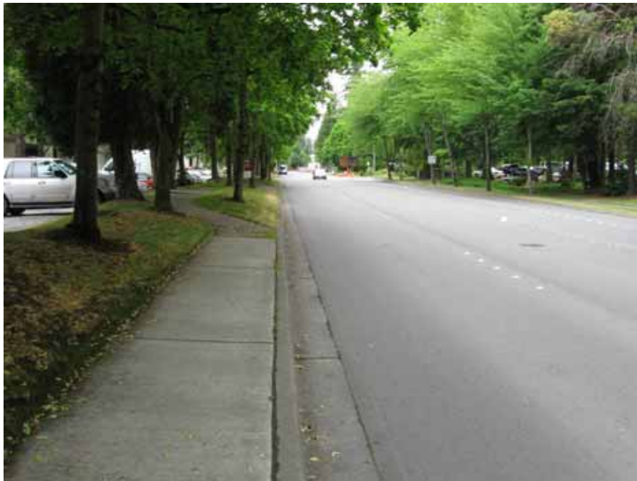
Photo #13—152 nd Avenue NE. Facing north.
