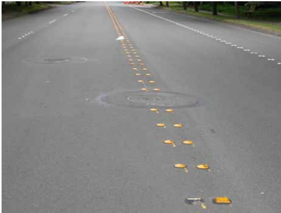
Photo #15—152 nd Avenue NE, facing north.
