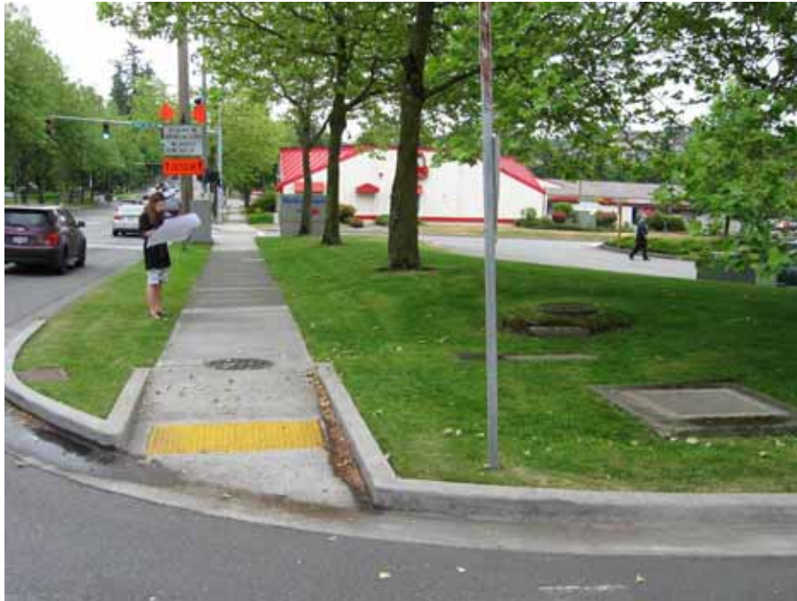
Photo #3—Critical conveyance invert location #4, Southeast corner of NE 24 th Street and 151 st Place NE. Facing east.
